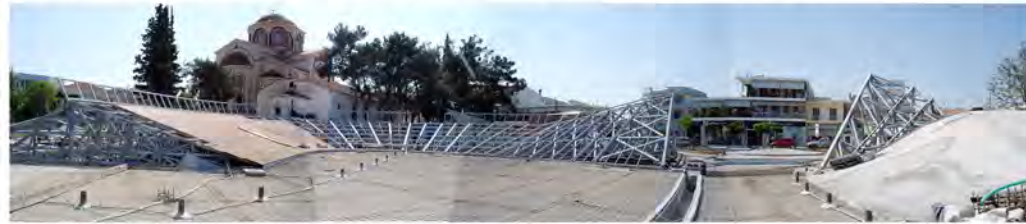
Figures 7,8 The metallic space frames as components derived from the cross-sections of the shape
